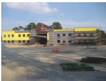
Sentara St. Luke's is scheduled to open in January 2010.
